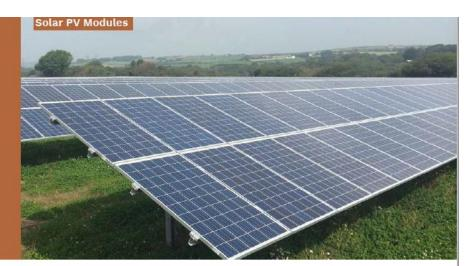
The areas marked as 'developable' will include solar photovoltaic (PV) modules that will convert sunlight into electrical current. We are proposing that each solar module will be approximately up to 2.5m long and 1.3m wide. The modules will each consist of a series of PV cells beneath a layer of glass. Each module will make up a single solar panel.
