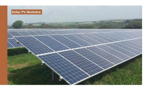
The areas marked as 'developable' will include solar photovoltaic (PV) modules that will convert sunlight into electrical current. We are proposing that each solar module will be approximately up to 2.5m long and 1.3m wide. The modules will each consist of a series of PV cells beneath a layer of glass. Each module will make up a single solar panel.
